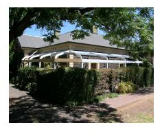
The new verandah frame incorporated bullnose shaped rafters, and intermediate purlins. The rafters and purlins provide support for the bullnose roofing. These was required because the verandah width exceeded the 1800 mm nominal maximum width for bullnose verandahs without rafter / purlin support. The additional support was also desirable because the roof will be accessed regularly for gutter cleaning.
